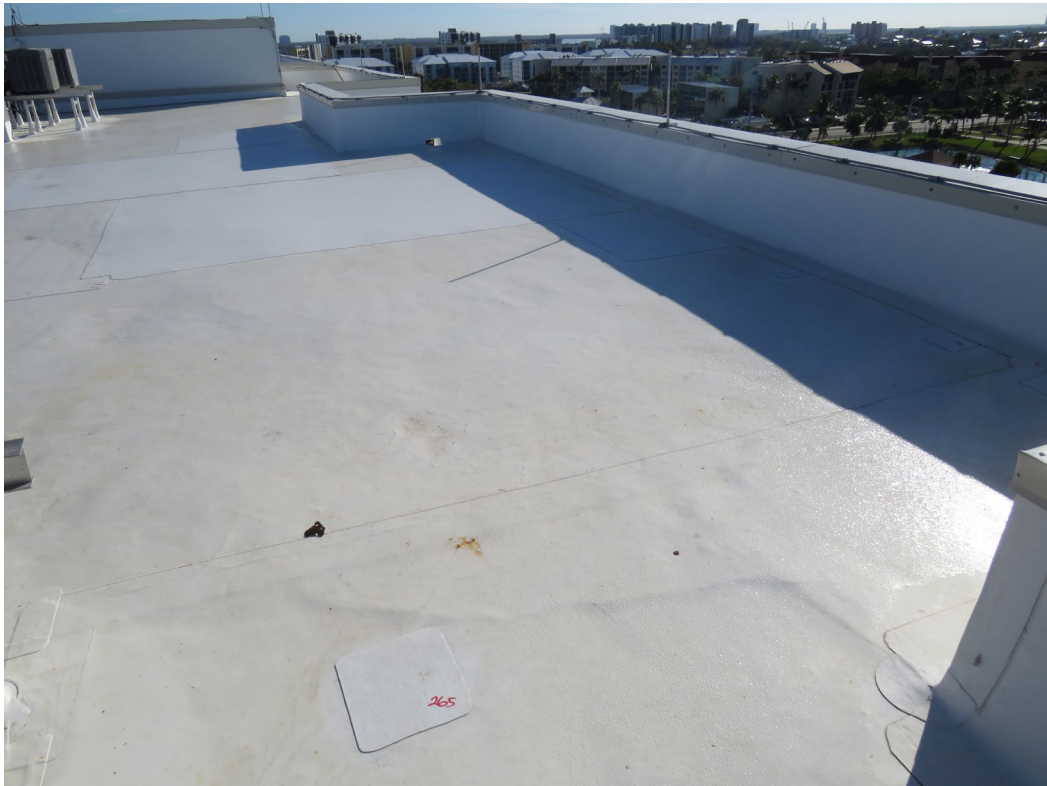
Photo 6, Overall view of TPO roof system.
