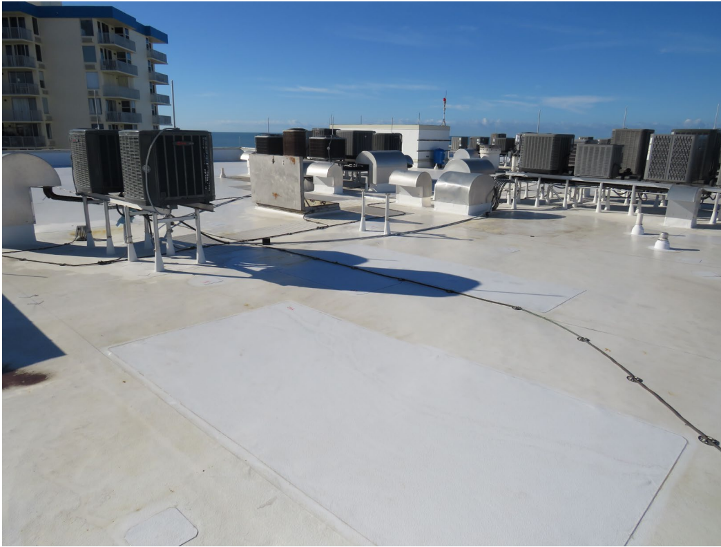
Photo 5, Overall view of TPO roof system.
