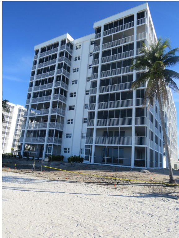
Photo 4, View of West Elevation.
