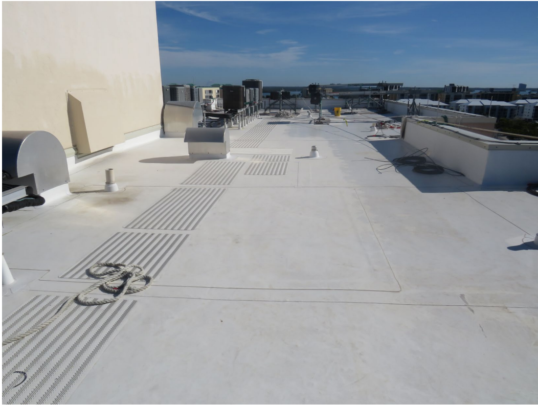
Photo 5, Overall view of TPO roof system.
