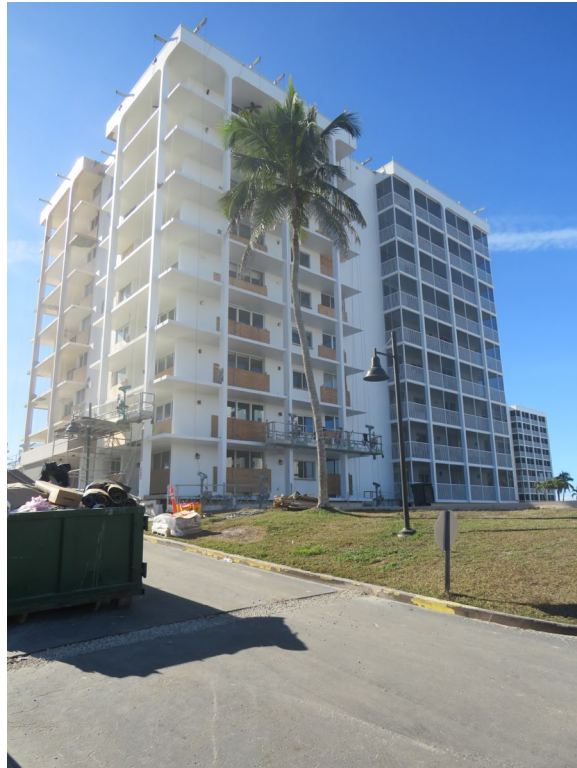
Photo 4, View of North Elevation.
