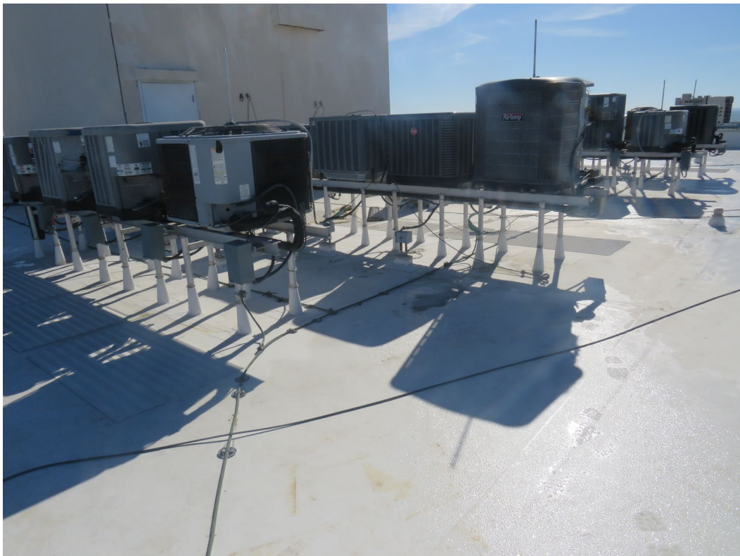
Photo 6, Overall view of TPO roof system.
